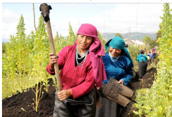
Quichua women dig pipe trench for their community water system
