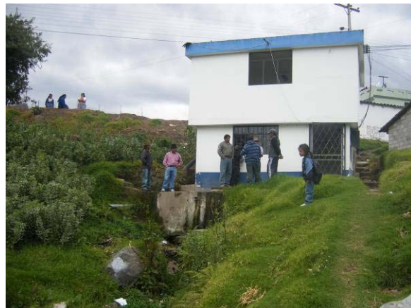
Peguche pump station and adjacent spring collector
