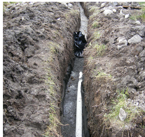
Figure no. 5 Trench Collector under construction
